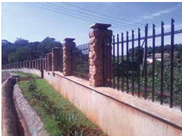
Figure 5. Migaa Masonry Wall with palisades.
